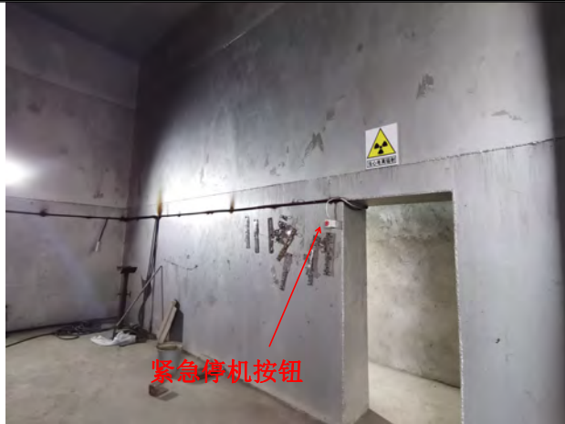
曝光室内西墙紧急停机按钮
